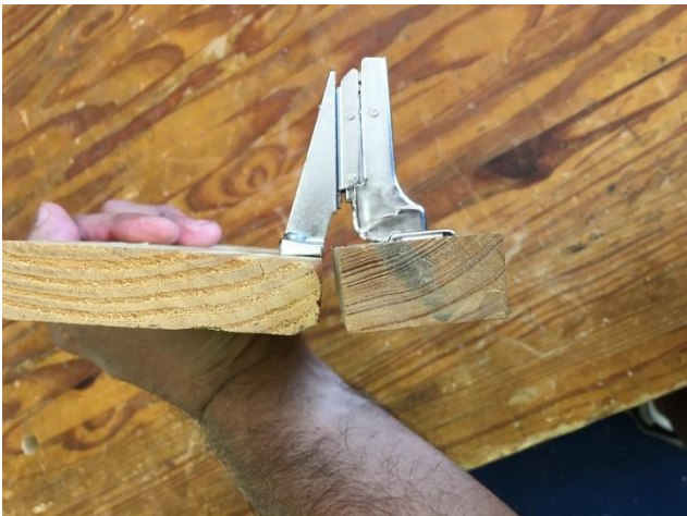
Stile appears to be cocked into cabinet – won't adjust flush
